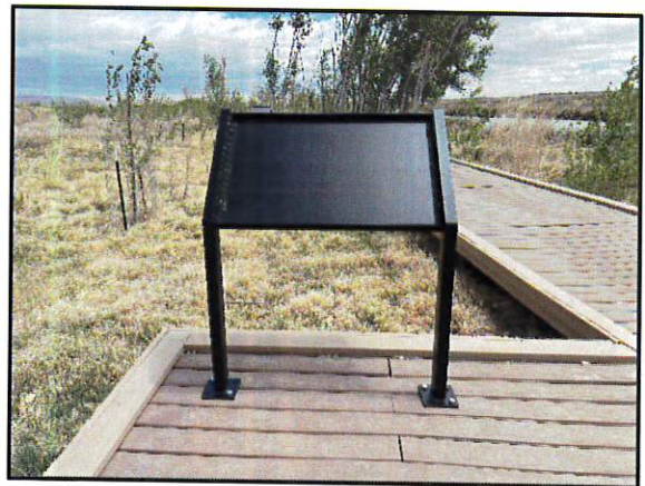
Figure 4. Installed Framework at Cottonwood Day-Use Area
