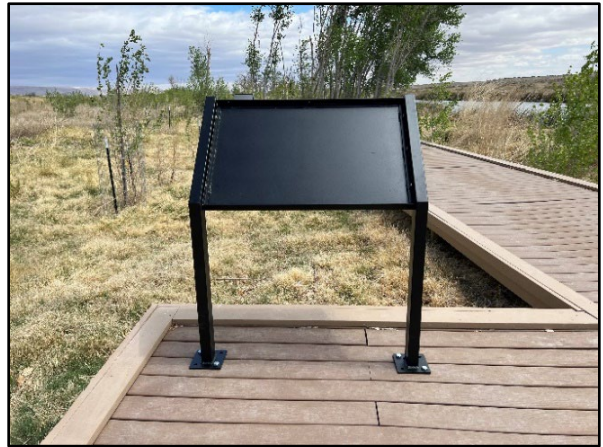
Figure 4. Installed Framework at Cottonwood Day-Use Area
