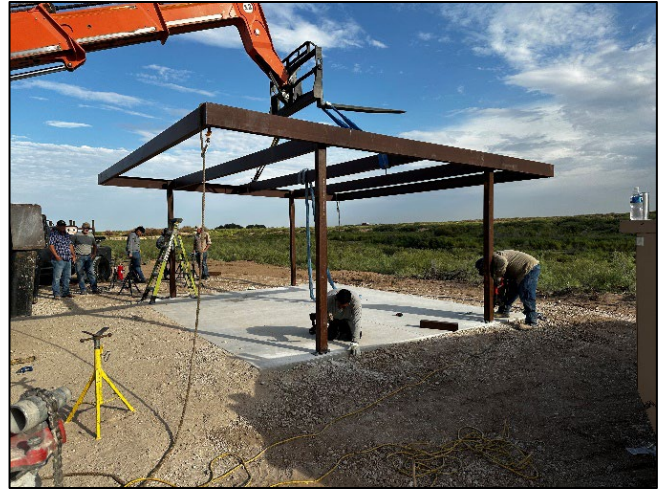
Figure 8. Industry partners installing shade shelters at Six-Mile Dam Improvement Project.
